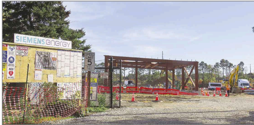
Site of the Sunrise Wind power station in Holtsville; Trump's executive order threatens offshore wind.
